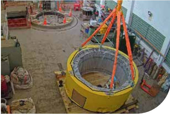
Unpacking new stator, the stationary part of a rotary system, at Waipori 4 station
